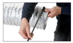
3. Pull the cable tie completely through the clip until it stops.
